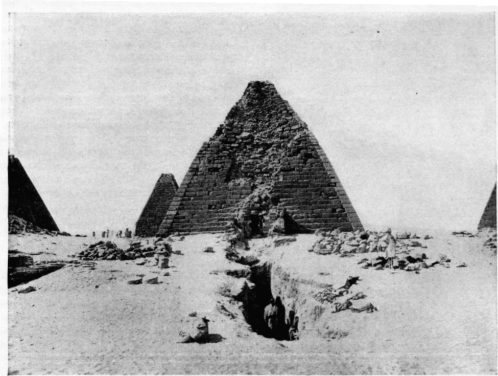
Fig. 2. Pyramid IV. Stairway and Chapel, looking west
