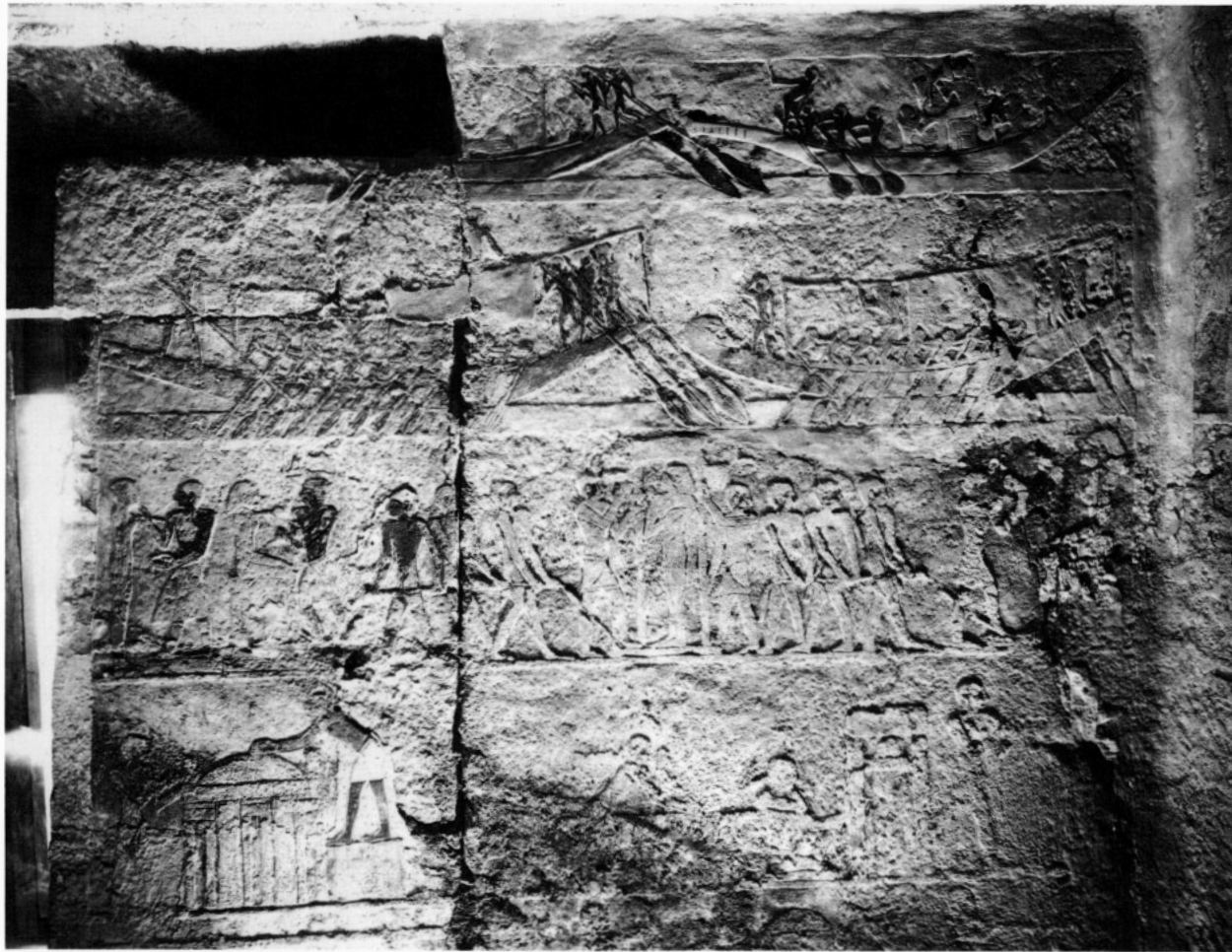
a. Main Room, East Wall, South, (7), Top
