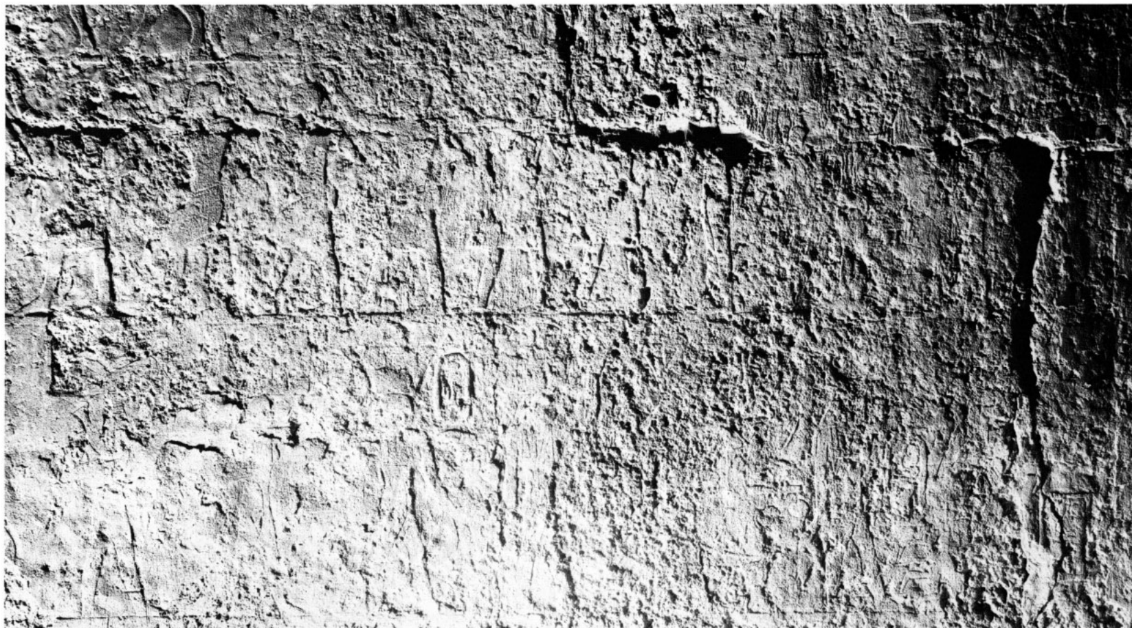
a. East wall, lower part of southern section
