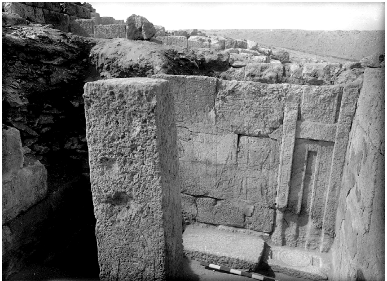
104b. 2098: pillar and west wall from east. The northern false door and its offering table are at right; the southern false door (behind the pillar) was removed in antiquity (a 8103)
