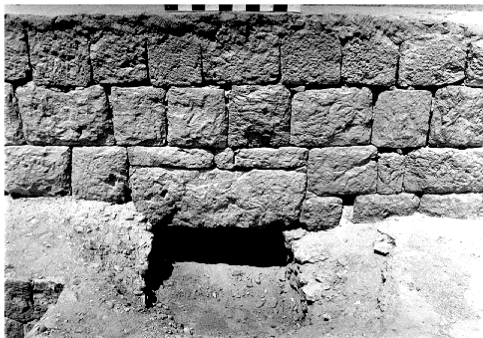
40d. 2091: east face wall supporting the corridor roofing, which was constructed over the reduced mastaba 2089, and had to bridge shaft 2089 b. The actual bridge was an unusually large block; three smaller blocks were laid above it to even the coursing (rg 10-13, 1989)
