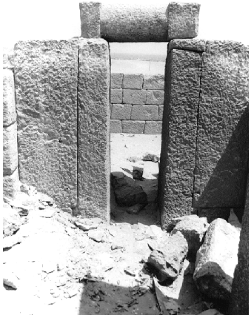
84a. 2097: doorway set between serdabs 2 and 3, leading from 2092+2093 courtyard into courtyard south of 2097. The direction of the drum lintel implies that it was an entrance to 2097 rather than 2092+2093, as does the elegant symmetrical stonework on this face. The large blocks behind the jambs rest on a lower course and a slight horizontal extension at the base of each jamb (amr, 1990)
