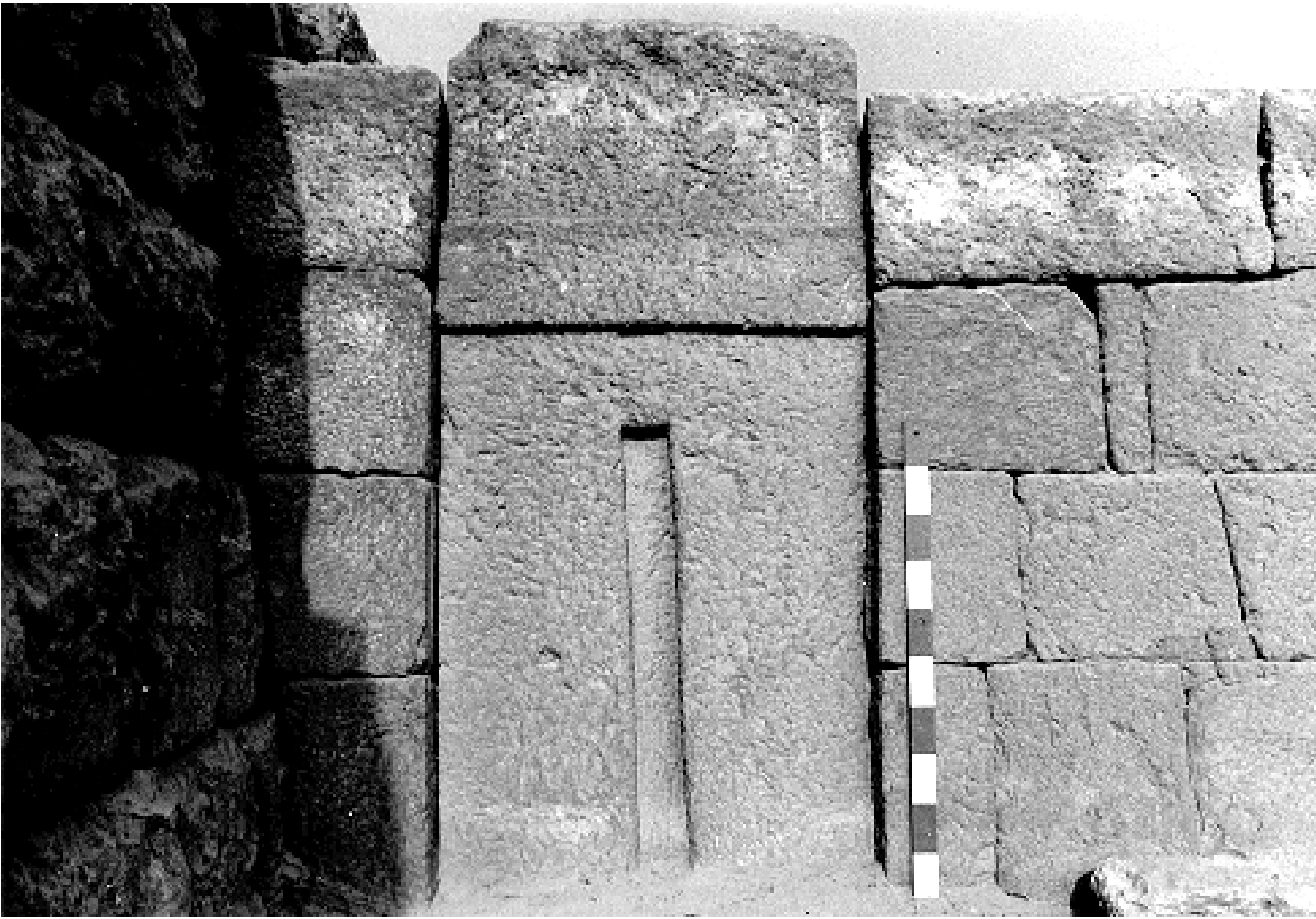
98a. 2097': undecorated false door at south end of east face (rg 7-4, 1989)
