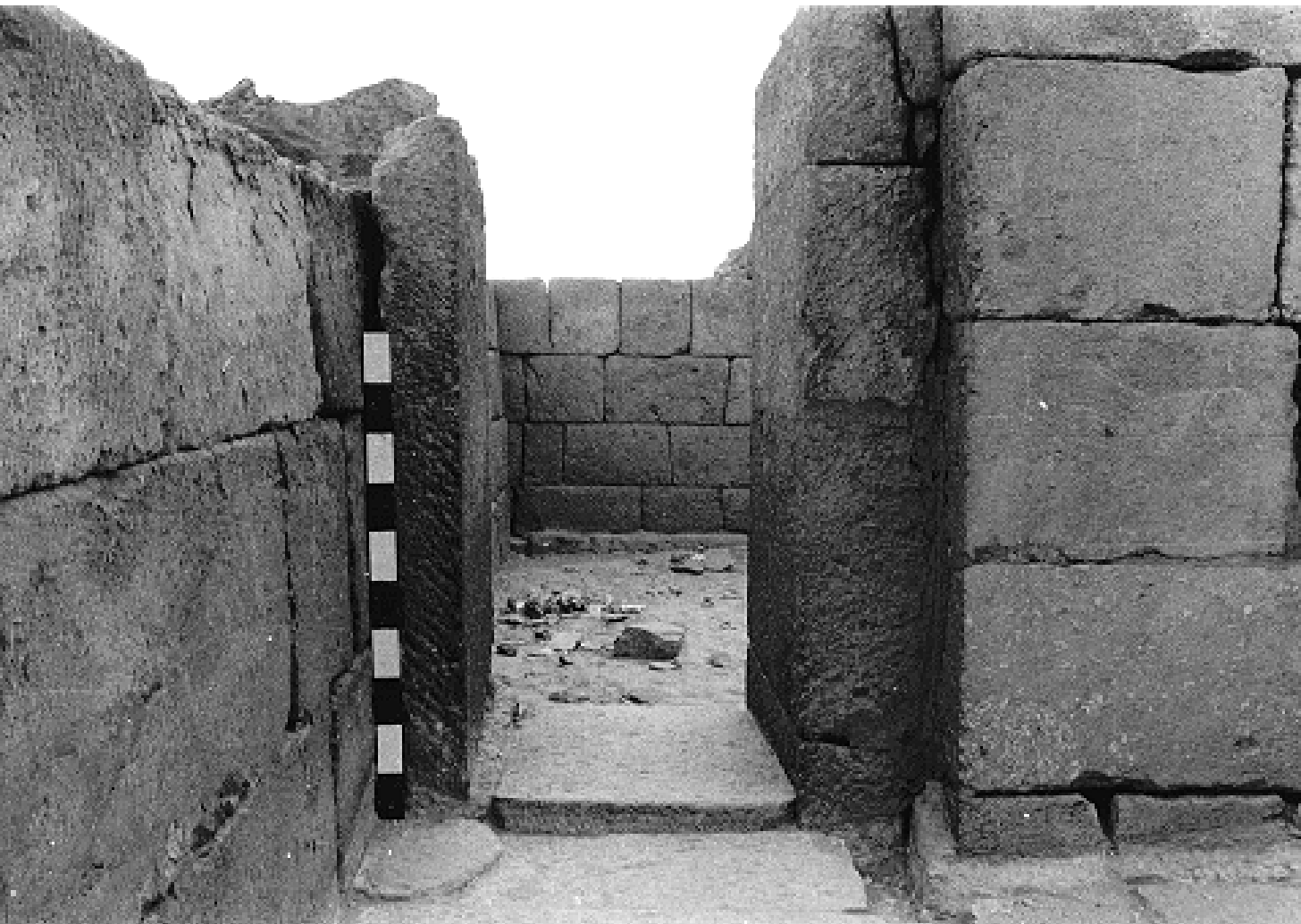
86b. 2097: door from chapel to courtyard. Beneath the scale stick is a raised round area which was perhaps intended to hold a door pivot, although the hole was never cut. To the right can be seen the "scar" left at the base of a wall when a floor block is removed (rg 6-15, 1989)
