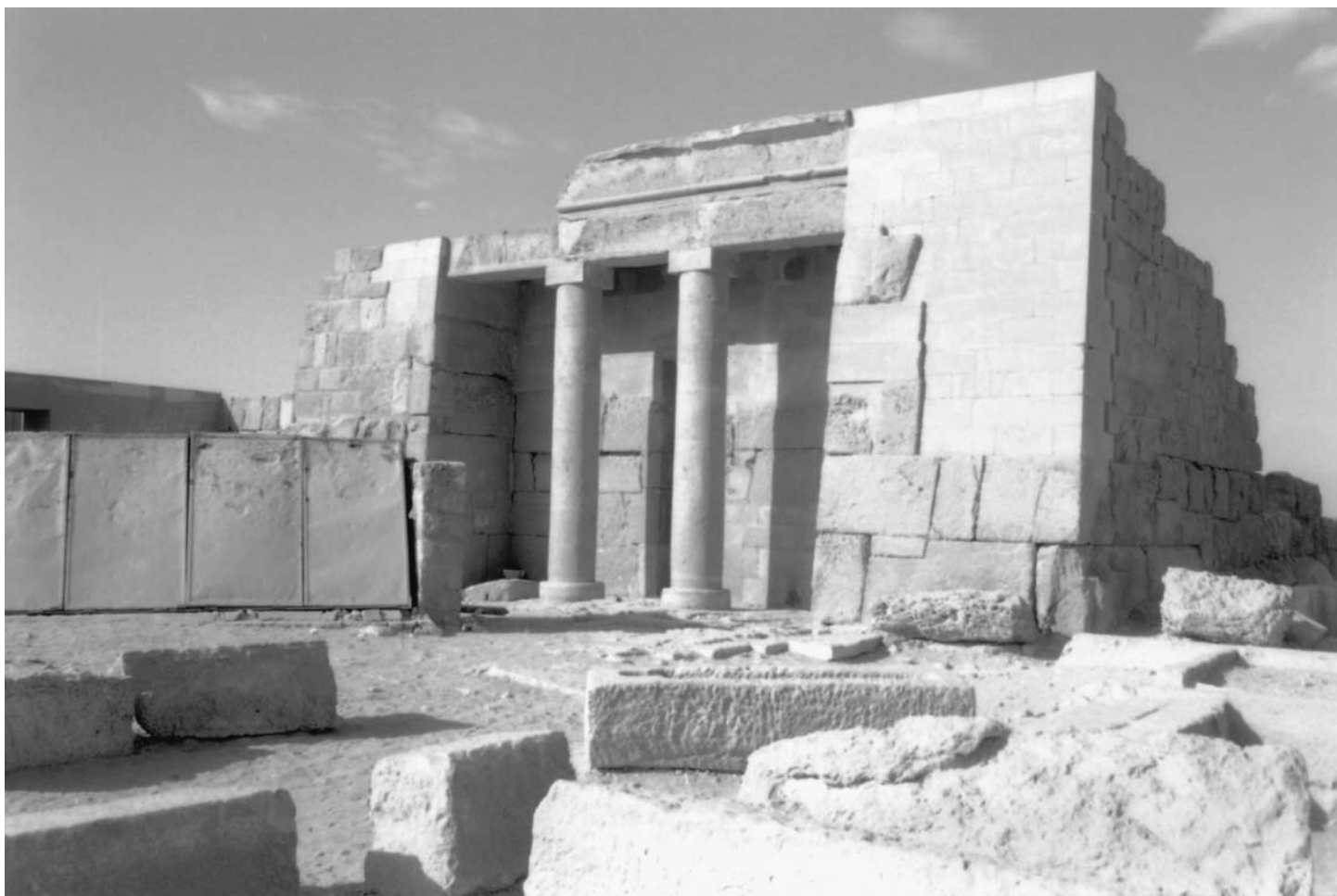
103a. Senedjemib Mehi (G 2378), reconstructed facade with light boxes of Sound and Light at left, looking northwest. December 1993. Edward Brovarski
