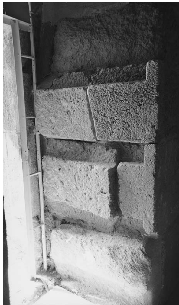
117c. Senedjemib Mehi (G 2378), Room II, inner west entrance thickness for battens on back of wooden door. February 1999. Bradford M. Endicott E 26-23
