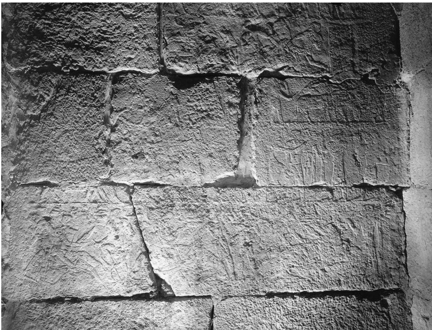
114b. Senedjemib Mehi (G 2378), Room II, west wall, lower section. 13 March 1931. HU-BMFA Exp. Ph. A 6365
