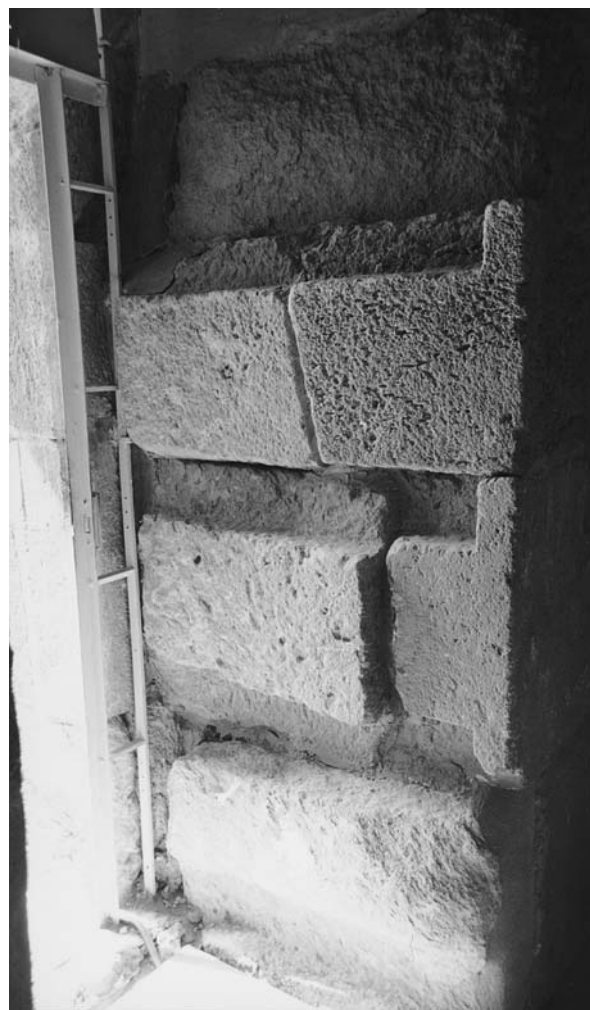
117c. Senedjemib Mehi (G 2378), Room II, inner west entrance thickness for battens on back of wooden door. February 1999. Bradford M. Endicott E 26-23
