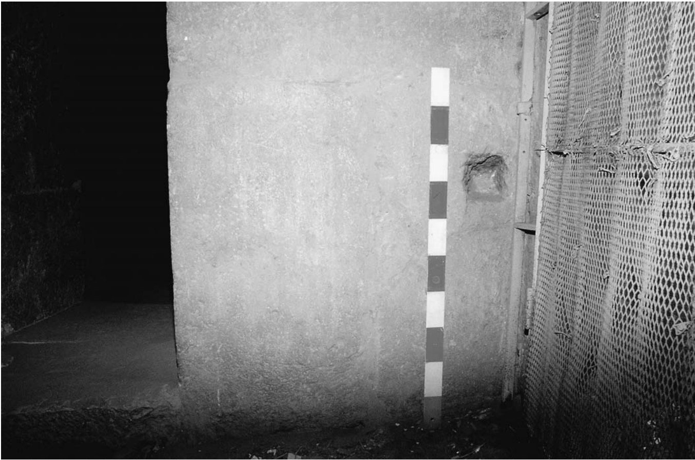
21a. Senedjemib Inti (G 2370), Room II, niche in north wall, looking northeast. 24 November 1993. Peter Der Manuelian 93.114.28
