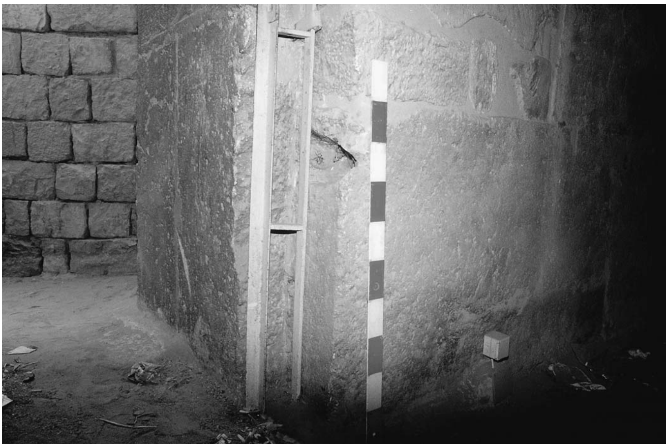
21b. Senedjemib Inti (G 2370), Room II, hole in north end of west wall, south of entrance, looking northeast. 24 November 1993. Peter Der Manuelian 93.114.29
