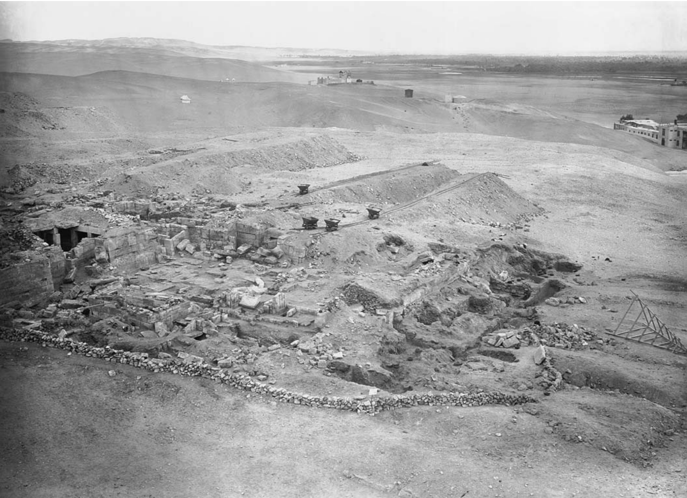
3a. Senedjemib Complex from the top of northwest corner of Great Pyramid, looking northwest. 11 December 1912. HU-BMFA Exp. Ph. A 810
