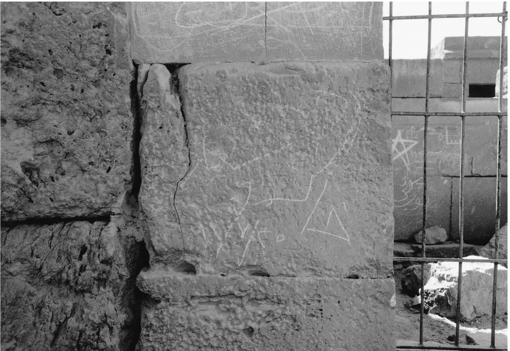
85b. Khnumenti (G 2374), facade, south of entrance. 30 March 1995. Edward Angelo, EA 1/22
