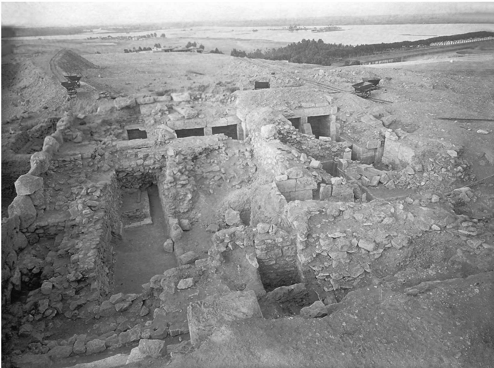
82a. Senedjemib Inti (G 2370), southwest corner of G 2370, looking north from photographic tower, with front wall of G 2371-72 at left, rear wall of G 2373 at right, and shafts G 2370 A and G 2373 A in middle foreground. 16 November 1912. HU-BMFA Exp. Ph. A 717
