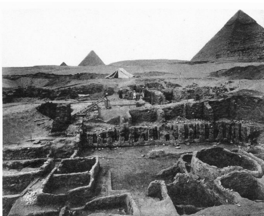
c. M. V. T., court, N. W. quarter, niched wall of court, looking west, February 17, 1910.
