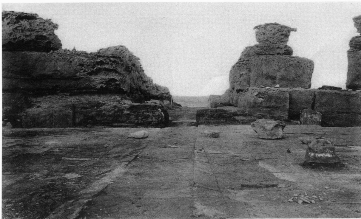
e. M. P. T., footway across court (5) and entrance corridor (3), looking east from center of court, June, 1907.
